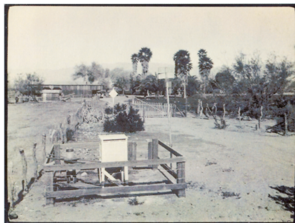
FIG. 2. The weather station at Greenland Ranch in 1926. The floor of the enclosure was reported to be 3.5 ft (1.1 m) above the ground in 1924. Courtesy of the Bancroft Library, University of California (BANC PIC 1978.027—ALB).
